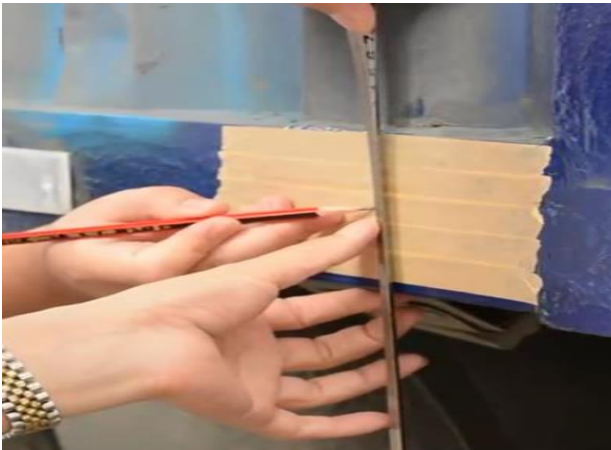
Measure the installation height drill holes
